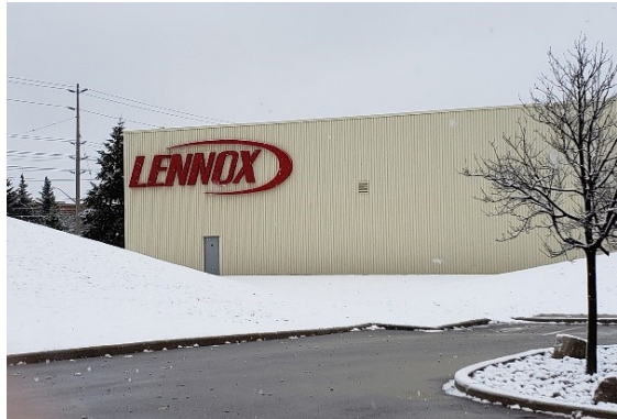
Brampton, Ontario Regional Distribution Centre
